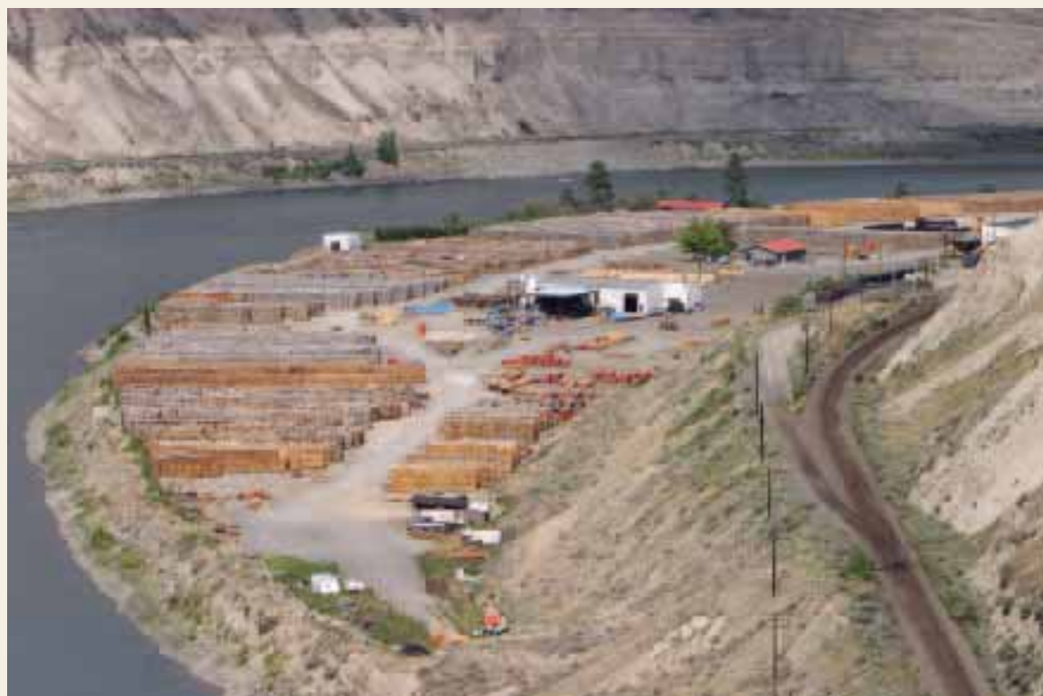
Ashcroft Treating Division
