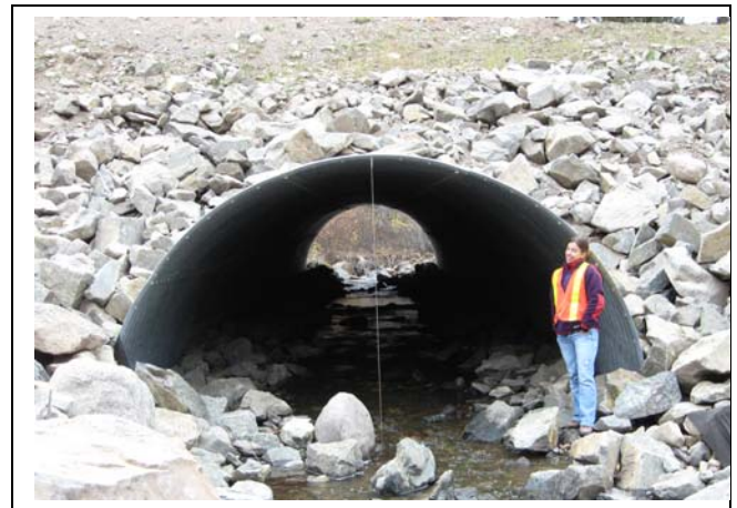
Photo #4: Restoring fish access to upstream habitat by replacing undersized culverts (left) with arch pipe culverts (right). Several of these projects were completed under the Forest Investment Account (FIA) program.
