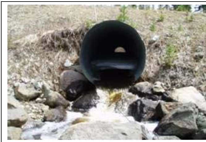
Photo #4: Restoring fish access to upstream habitat by replacing undersized culverts (left) with arch pipe culverts (right). Several of these projects were completed under the Forest Investment Account (FIA) program.
